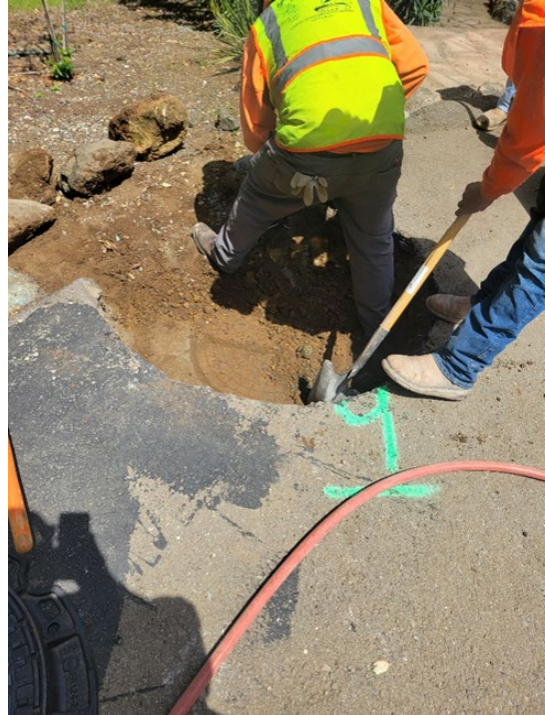
Excavating manhole cover at Bradford Circle
