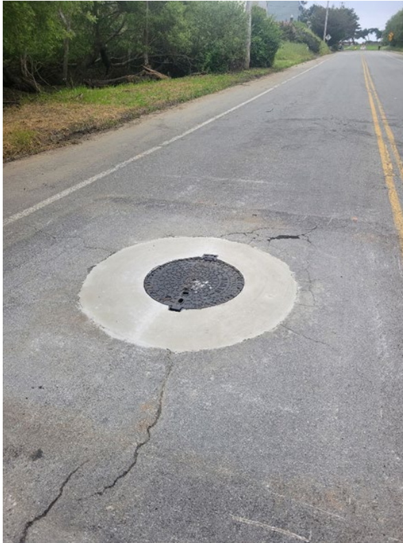
Replaced manhole ring and collar at
