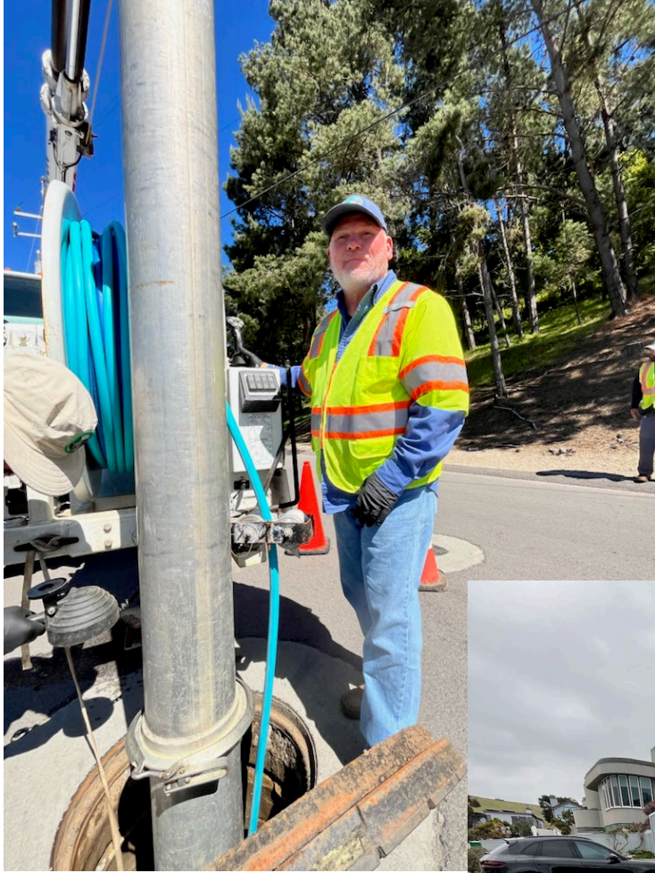
Tim, jetting and vac'ing
