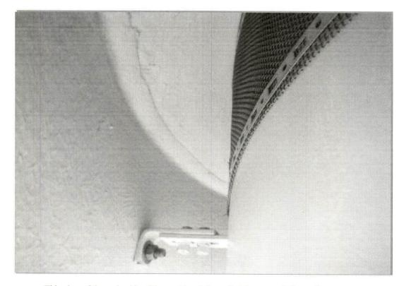
This view of the underside of the vent hood shows that the screen is in good condition and are free of corrosion.
