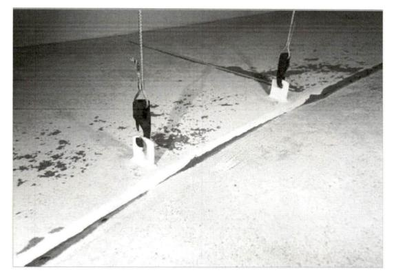
Level gage guide wires and attachment tabs on the interior bottom. Minor corrosion is present at the inaccessible area under the attachment hook. This is considered normal and acceptable.
