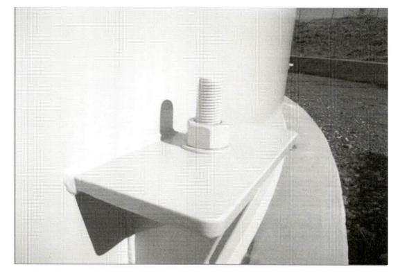
Tank exterior shell, chine and anchor. No corrosion or issues were noted.
