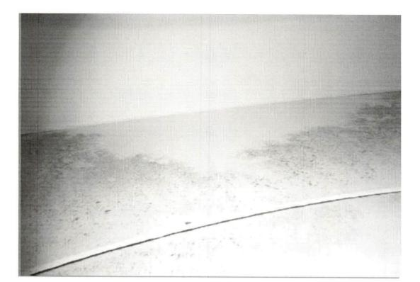
Lower shell and tank bottom. Coatings are in good condition in this zone with the exception of a few rust points that were repaired by the diver.
