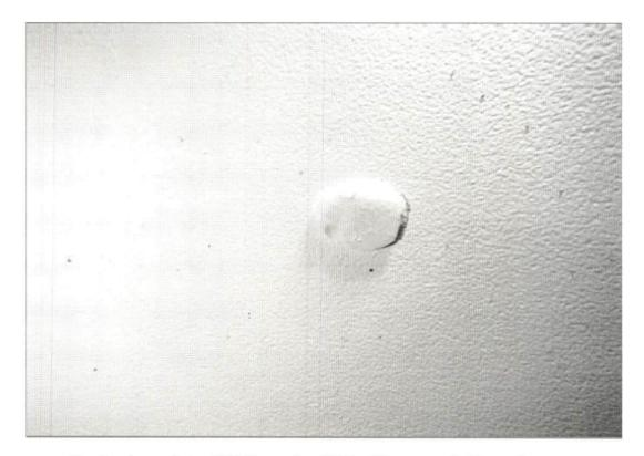
The diver has applied an NSF 61 compliant 100% solids epoxy and ATS proprietary cure barrier repair.
