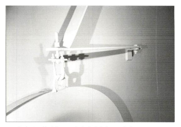
Interior view of the shell manway showing the davit where corrosion issues are most likely to occur. Some minor corrosion was present at inaccessible areas.
