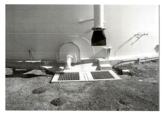
Exterior view of the flush clean-out, drain and overflow. Some minor corrosion is present.
