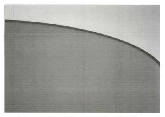
This view represents the typical conditions on the upper shell and shell to roof joint. The upper shell is in good condition with no corrosion points noted.
