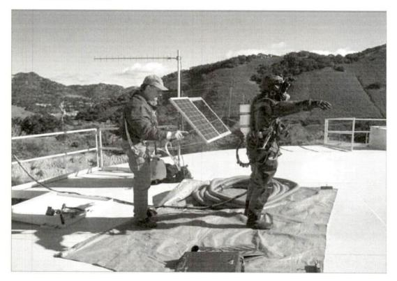
Diver and equipment are disinfected with the chlorine solution just prior to entry. This procedure is pursuant to AWWA disinfection standards for potable water diving (stock photo).
