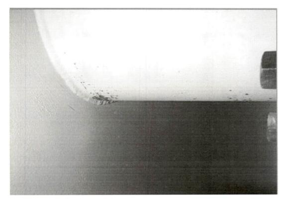
Underside of inlet/outlet with corrosion point which was subsequently repaired by the diver.
