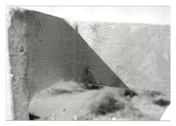
Several of the "cold galv." field repairs of the field welds on the hot dip galvanized parts have rusting.
