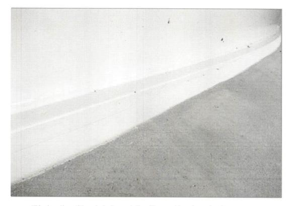
This close view of the exterior lower shell and bottom chime shows that the caulking is in good condition and the seal is effectively protecting the chime.
