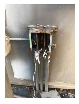
Figure 2 New electrical pull box
