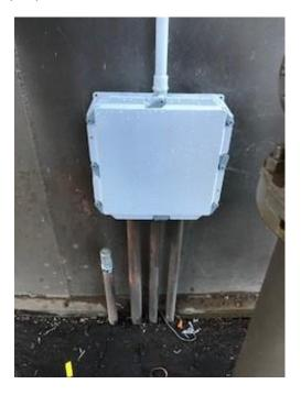
Figure 3 Rusted electrical pull box
