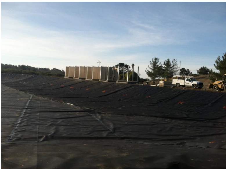
Mechanical Evaporator Sound Enclosures being installed
