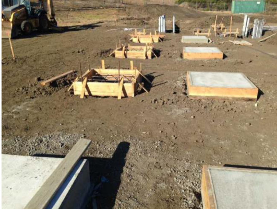
Forms Set for Shipping Container Support
