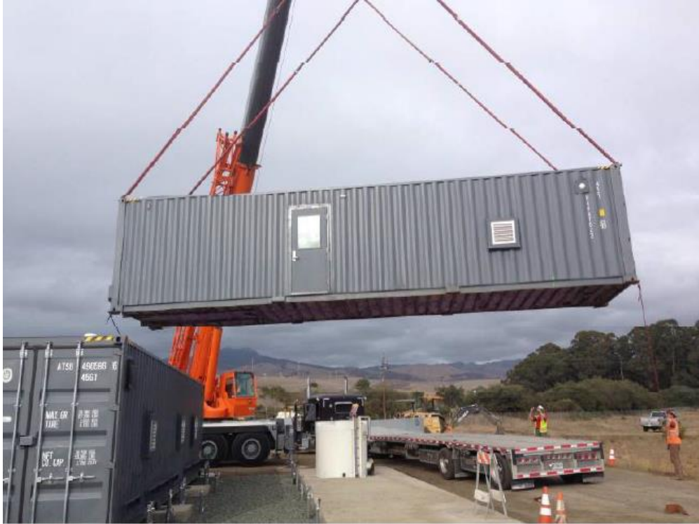
Shipping container unit In process of being set into position
