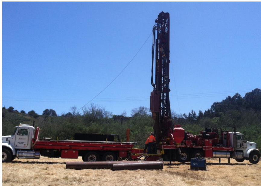
Re-injection Well Installation
