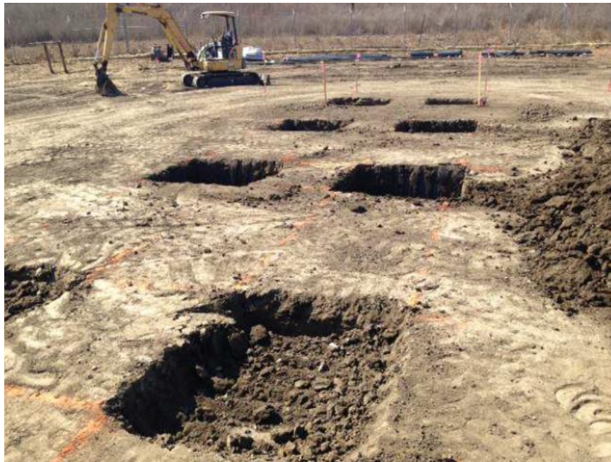
Excavation into Re-compacted Area for Shipping Container Support
