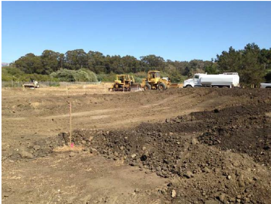
Initial Clearing & Grubbing at Evaporation Pond
