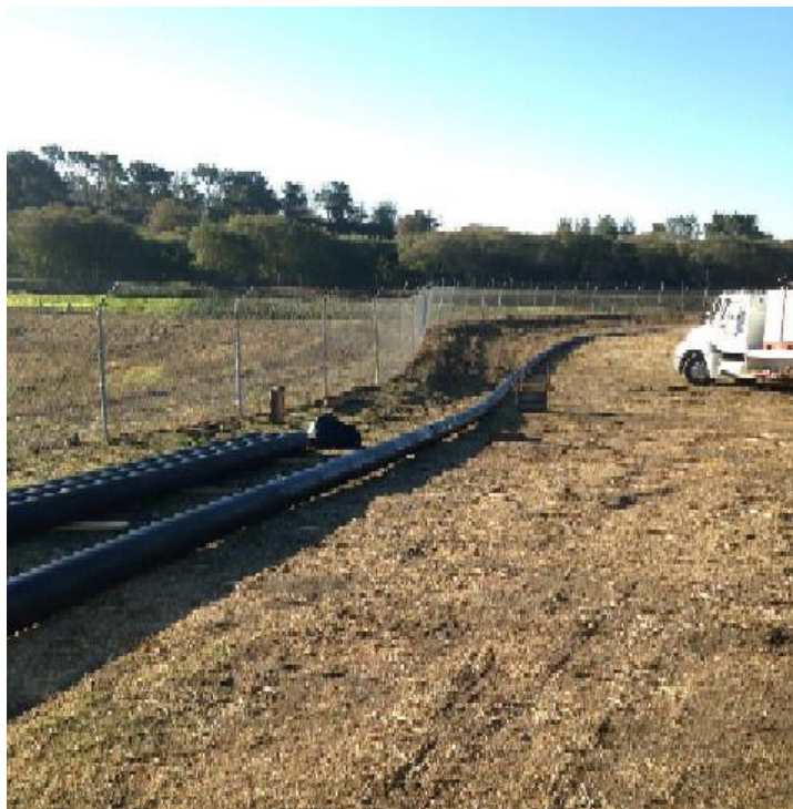
HDPE Pipeline between AWTP and Evaporation Basin
