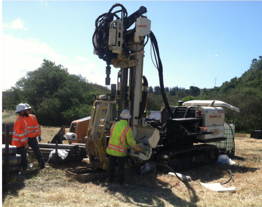
Monitoring Well Installation
