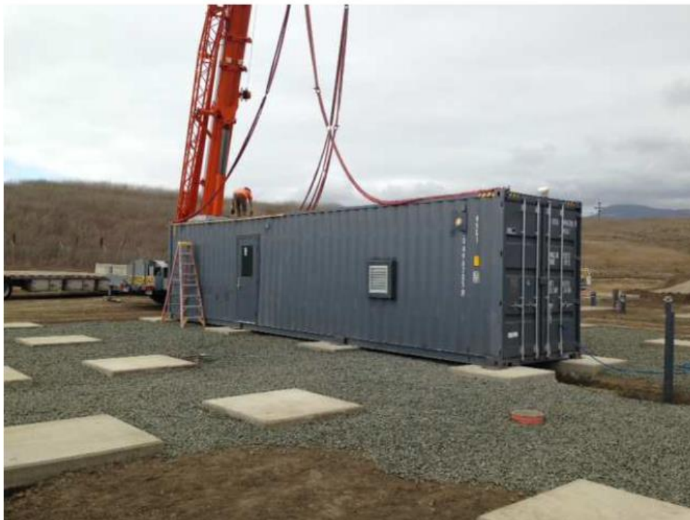
Shipping container set into position
