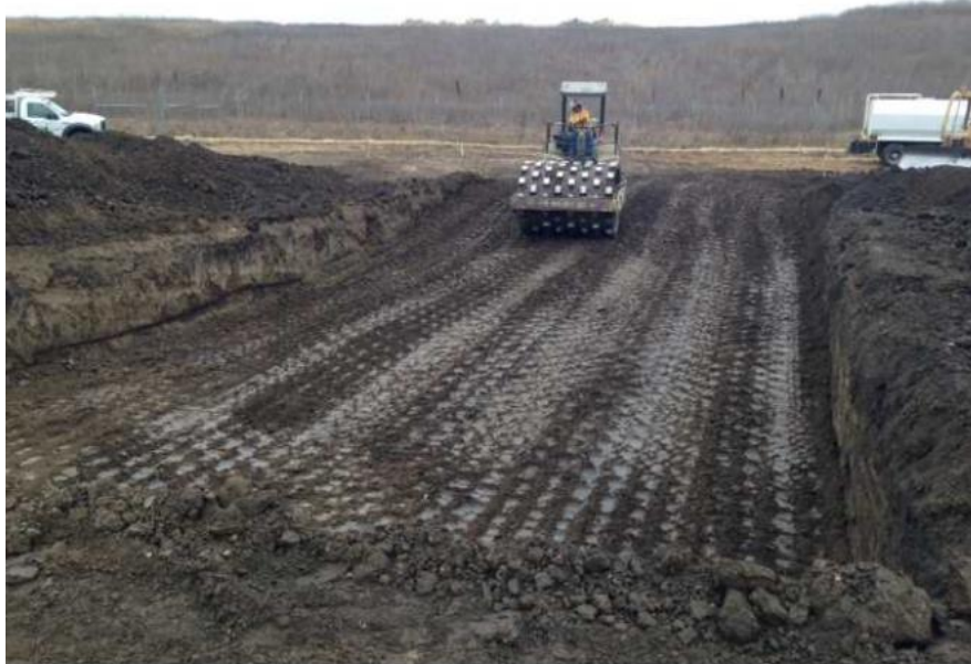
Re-compaction at the AWTP Site
