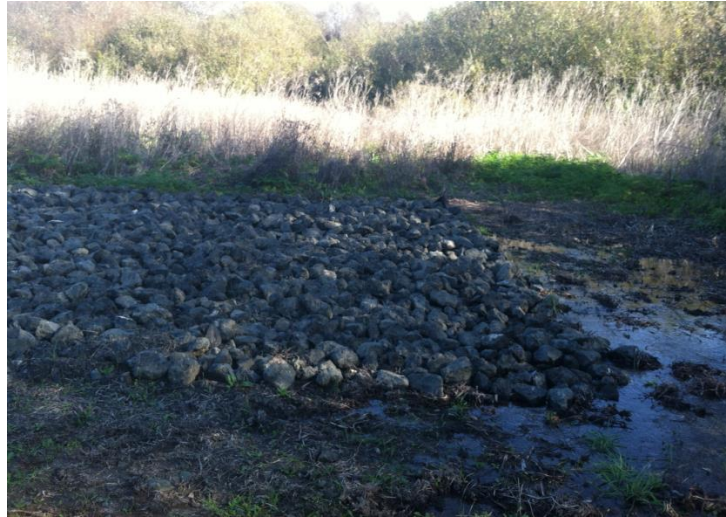
Lagoon Water Discharge Structure Outside of Tree Drip Line at Upper San Simeon Creek lagoon
