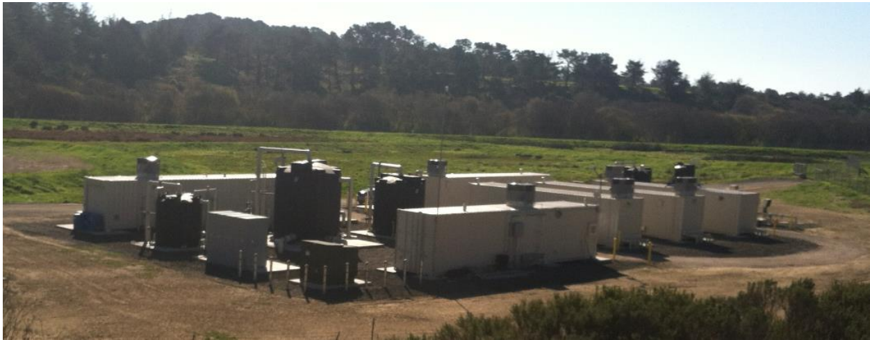
View of Completed AWTP
