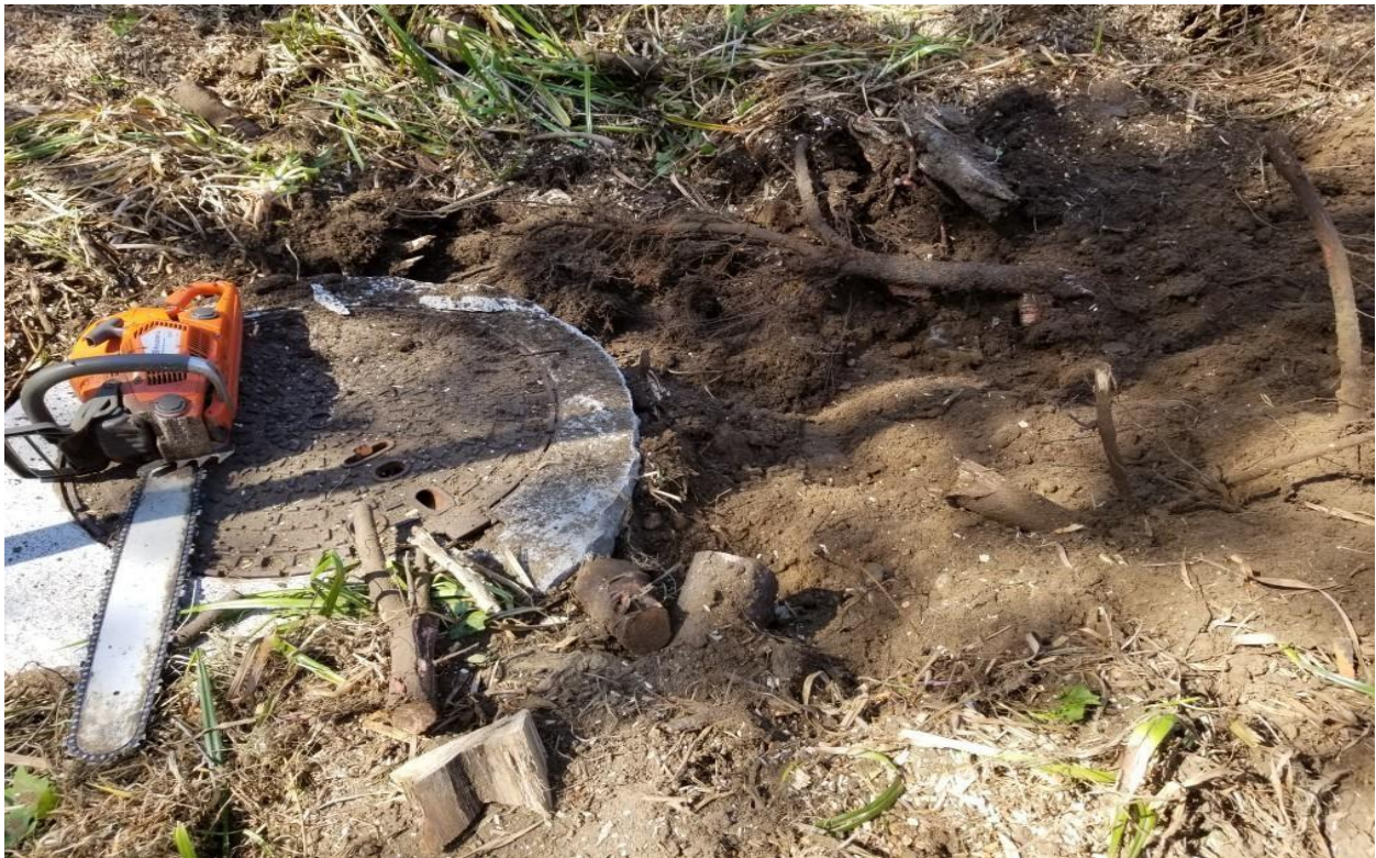
Figure 3 Manhole repair due to root intrusion
