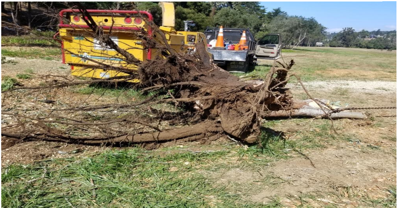
Figure 4 Removed segment of tree during repair
