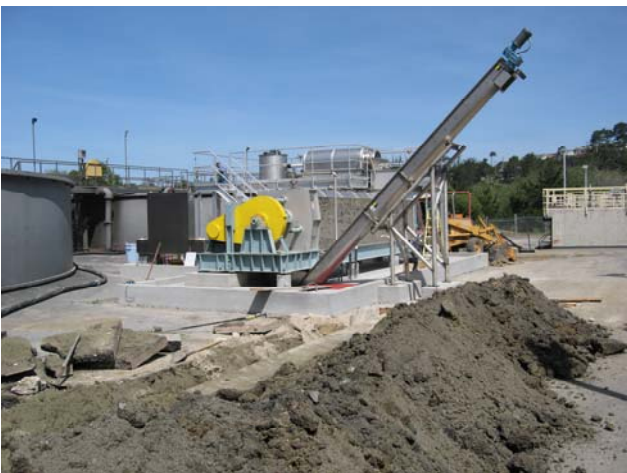
Installing Screw Conveyor Pit Drain
