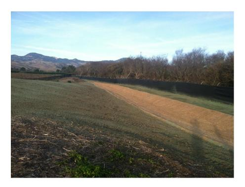
12/7/2017 View looking south along the new drainage swale that is located to the east of the impoundment. Recently hydro-seeded areas show as green areas. The eastern fencing shown to the right of the new swale was repaired during late summer/early fall of 2107.
