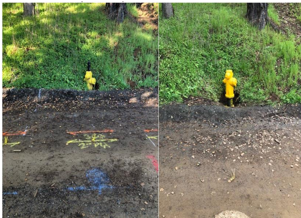
Figure 4 Sandown hydrant before (left) and after raising (right). Blue paint in before photo shows location of buried valve.
