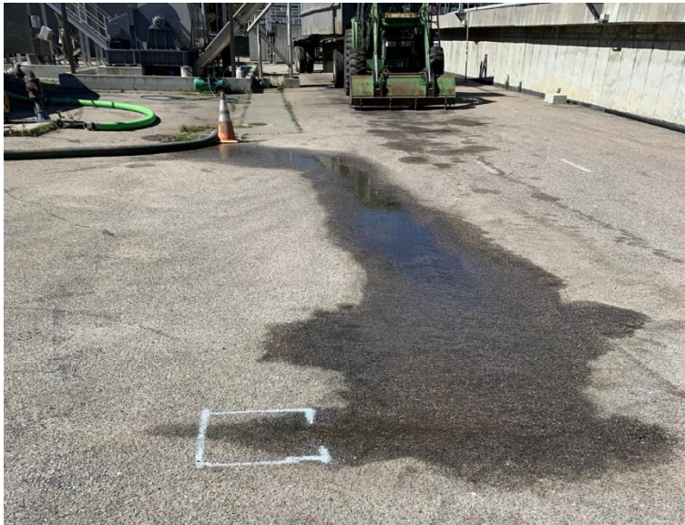
Figure 1 Leak at WWTP
