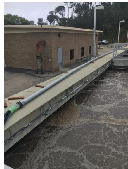
Figure 8: Aeration Basin and Blower Building
