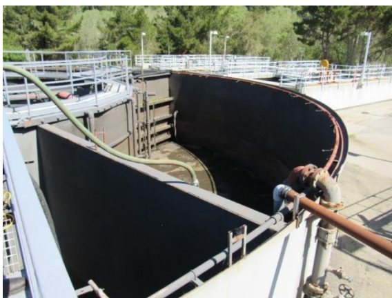
Figure 4: Existing South Clarifier (from south)
