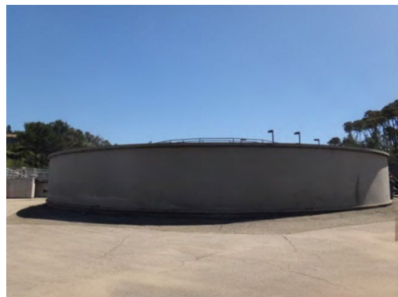
Figure 5: Existing South Clarifier (from west)
