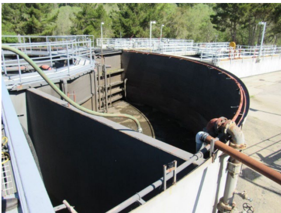
Figure 4: Existing South Clarifier (from south)
