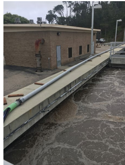
Figure 8: Aeration Basin and Blower Building
