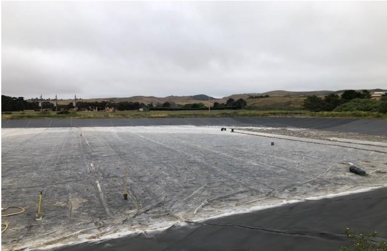
Figure 4 Basin June 10, 2019 (mid-removal of solids)
