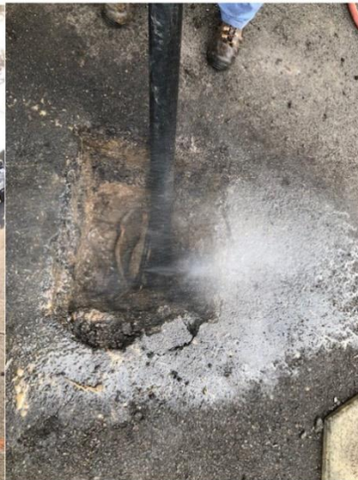
Figure 6 (Left) Ditchwitch at leak repair (Right) Excavated leak
