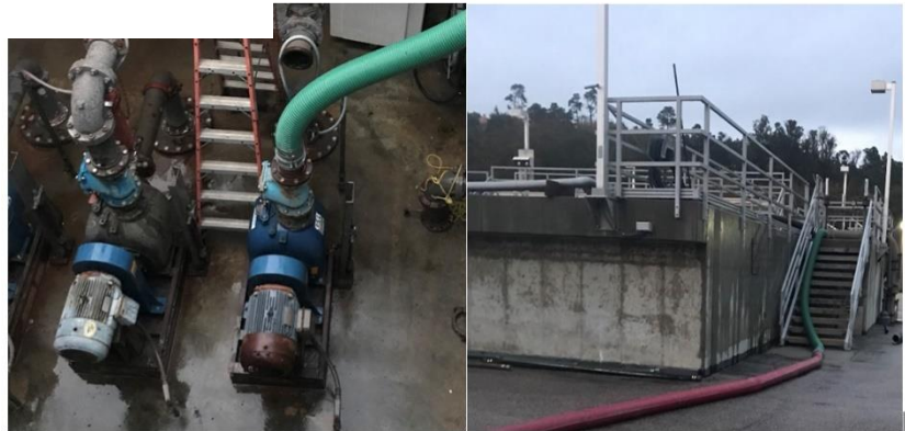
Figure 2 (Left) Influent Pump #1 (Right) Lay-flat hose running to the aeration basin
