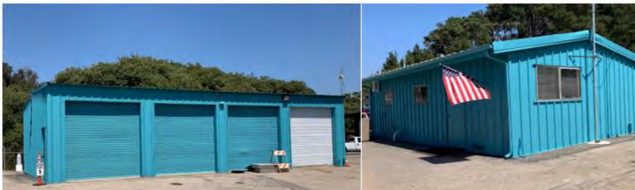
Figure 3 Shop and breakroom with fresh paint.
