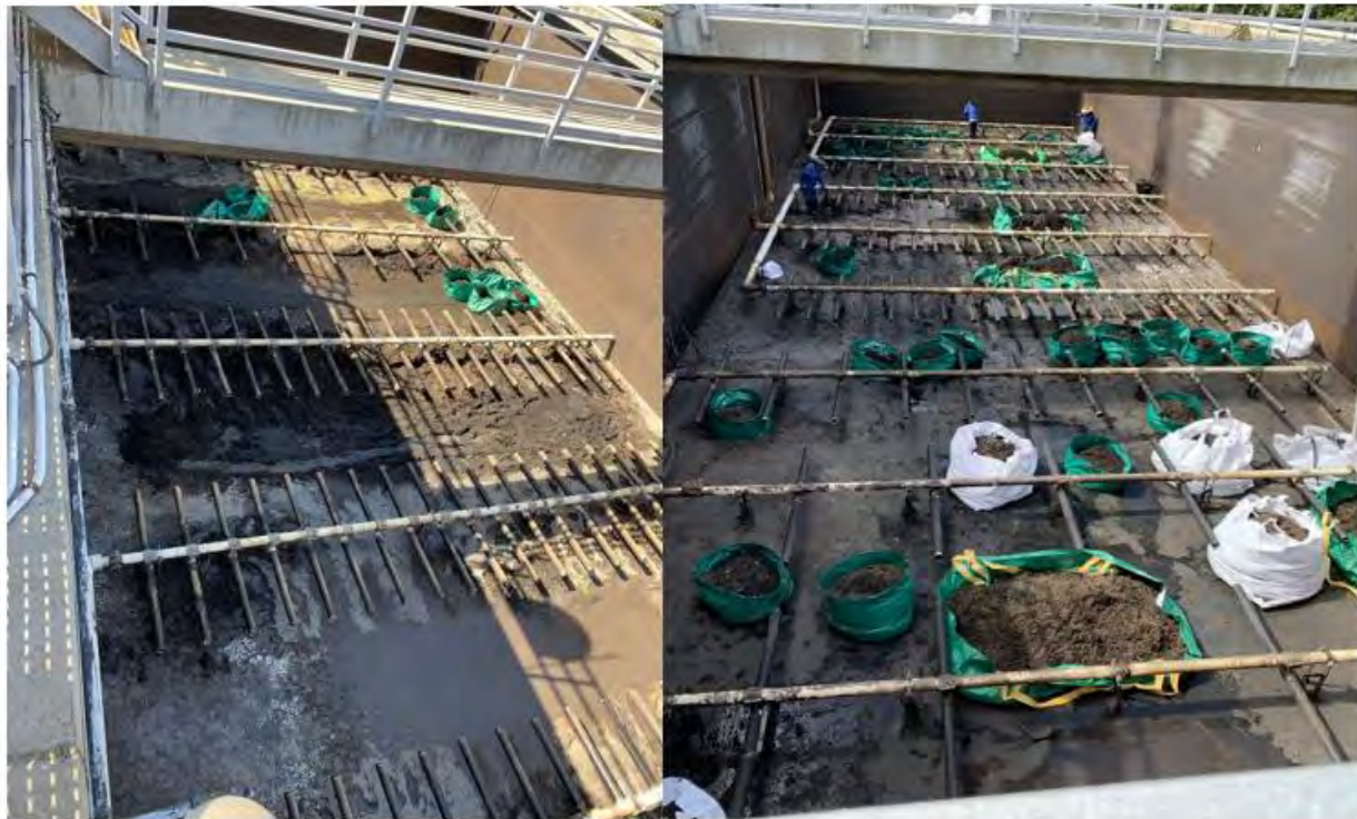
Figure 1 Aeration basin #2 drained and being cleaned
