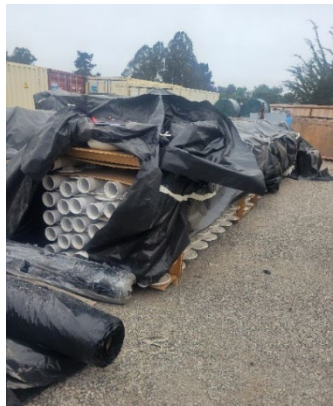
Air header piping for the aeration basins
