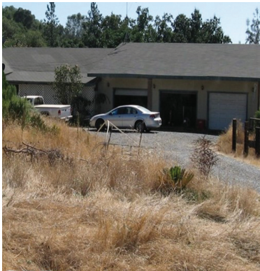
DEFENSIBLE SPACE NONCOMPLIANT
