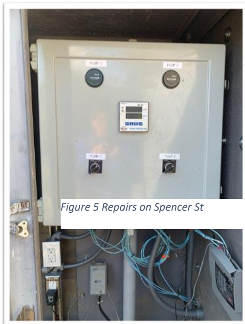
Figure 5 new controls at lift station B-1
