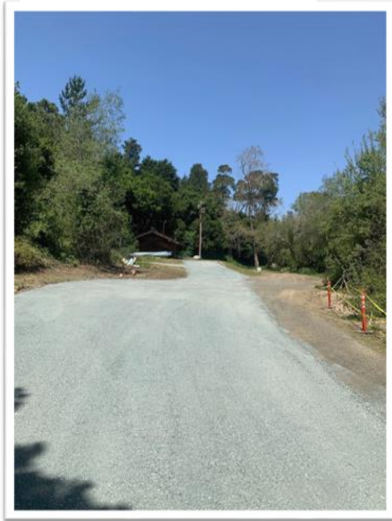
Figure 2 Lift Station B approach
