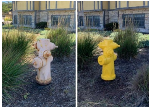
Figure C - Fire hydrant before (left) and after (right) CCSD maintenance
