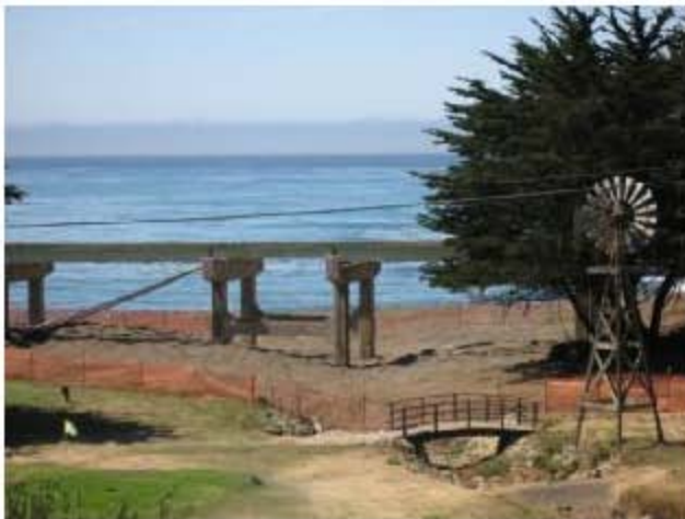
Leffingwell Bridge Deck Off August 25, 2008
