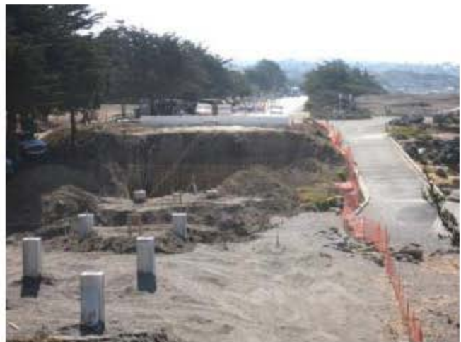
Leffingwell Bridge Deck Off September 17, 2008
