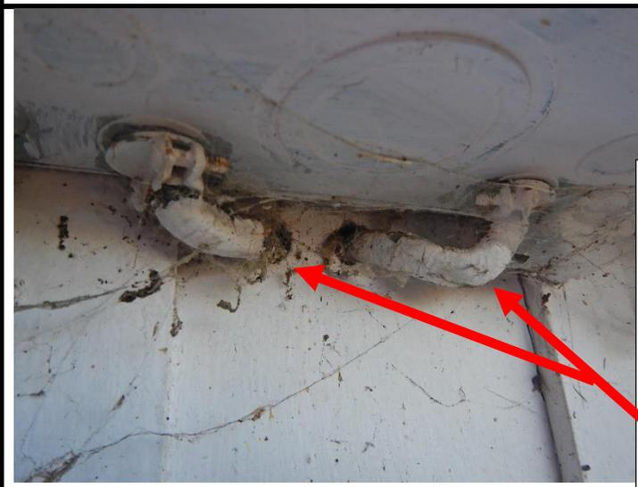
3 **Exposed electrical wiring or "Romex" found not installed to minimum standards subject to physical damage not in a conduit or raceway per standards. Safety Hazard: ON THE EXTERIOR AT THE MAIN ELECTRICAL PANELS.**
