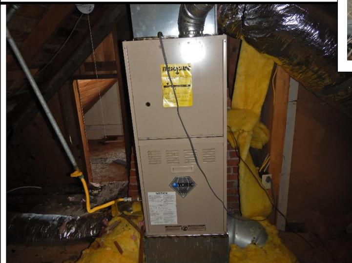
14 **Disclosure: The Heater located in the attic appears to be newer and looks to be in good condition. Unable to test due to the lack of gas and electric.**
