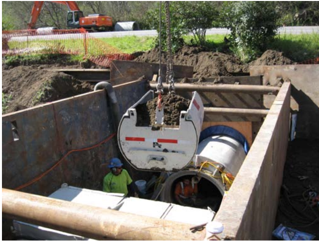
Boring machine and bucket under Highway 1
