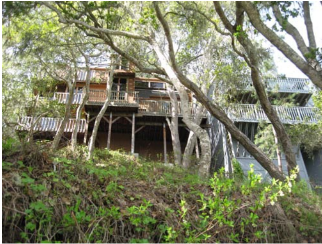
Extremely flammable homes on steep slopes
