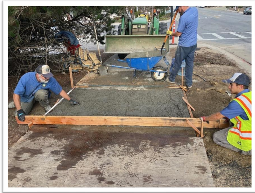
Water Systems Operators replacing the sidewalk on October 24
