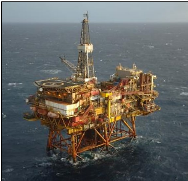
Figure 12. Photo of Brent Alpha prior to decommissioning in the North Sea (Shell 2020a)
