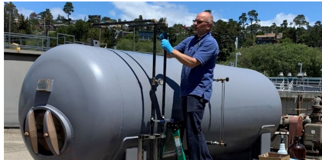
Figure B- Operator Toni Artho repairing effluent discharge surge tank
