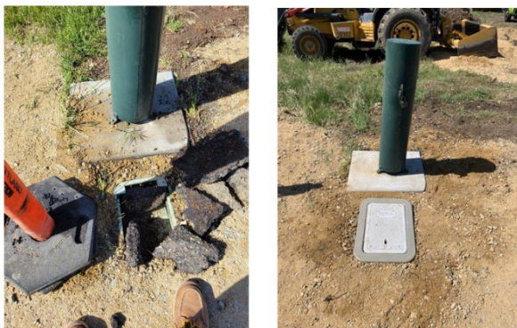
Figure A – valve box before (left) and after (right)
