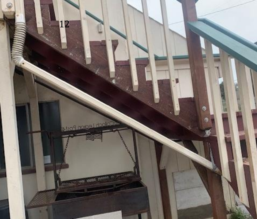
Vet's Hall Rotted posts, stair stringers and parts were replaced with pressure treated lumber.
