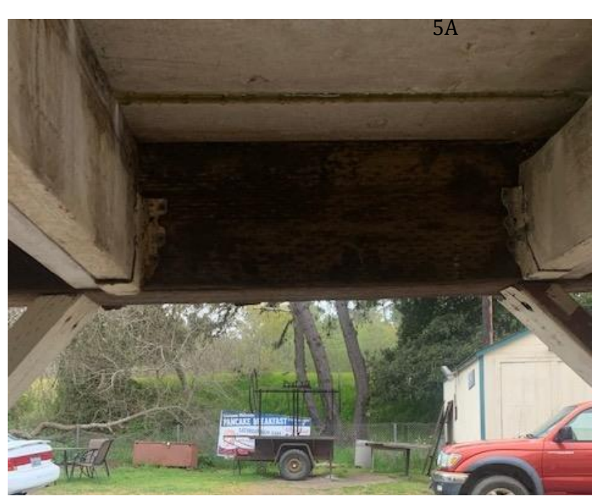
Vet's Hall Rotted posts, stair stringers and parts were replaced with pressure treated lumber.
