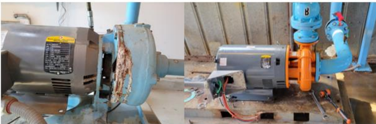
Figure D - Booster pump before (left) and after (right) repair
