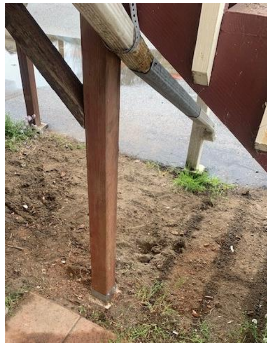
Vet's Hall Rotted posts, stair stringers and parts were replaced with pressure treated lumber.
