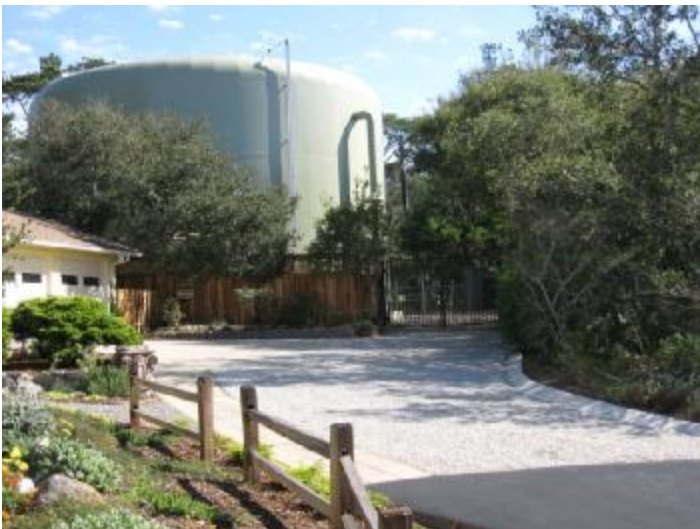
The New Pine Knolls Tanks
