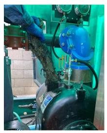
Figure 2 Lift Station Pump Maintenance - Clog Removal
