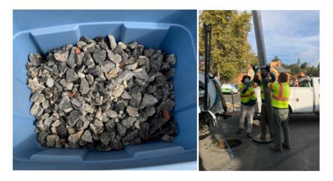
Figure 1 Debris cleared from lines (left) and staff clearing manhole with the Vactor Truck (right)
