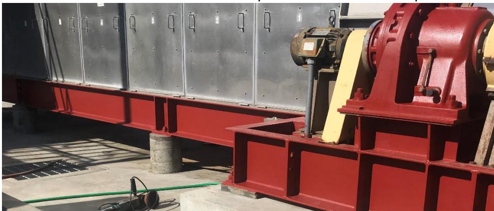
Figure 5 Sludge press with rust converter
