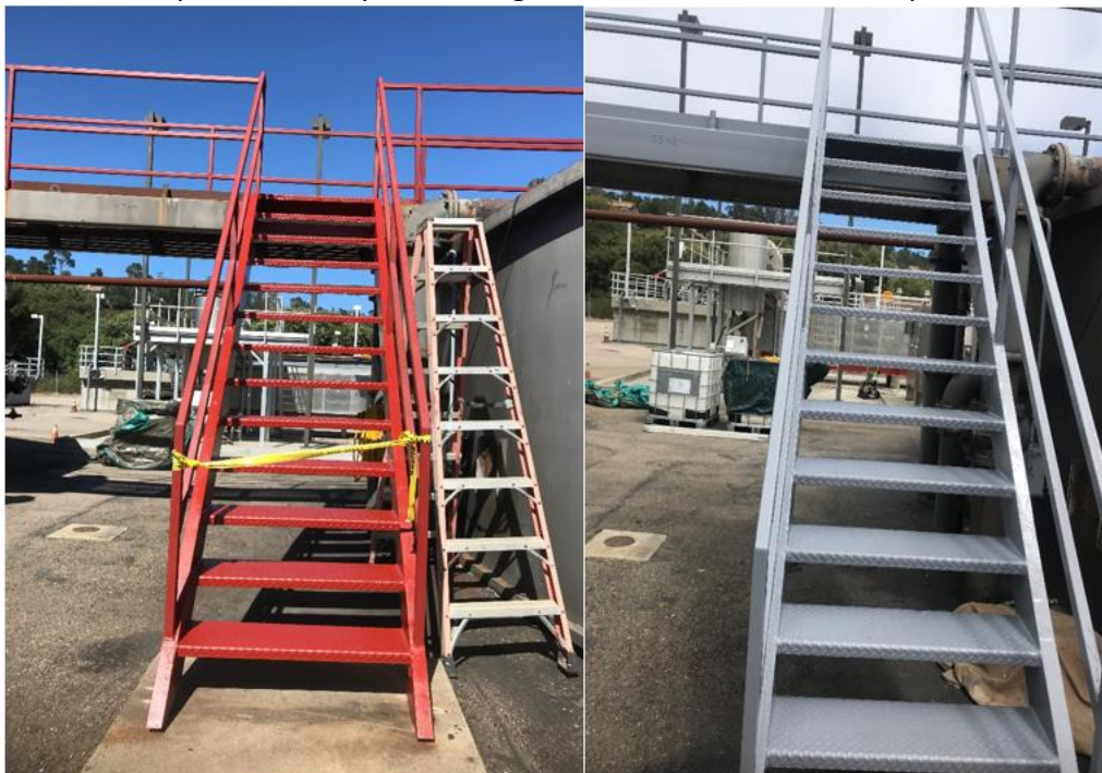
Figure 1 Freshly painted digester handrails with rust converter (left) and paint (right)
