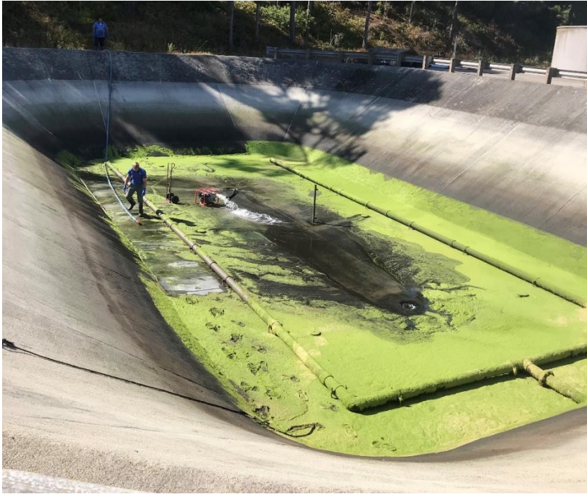
Figure 3 Effluent holding pond
