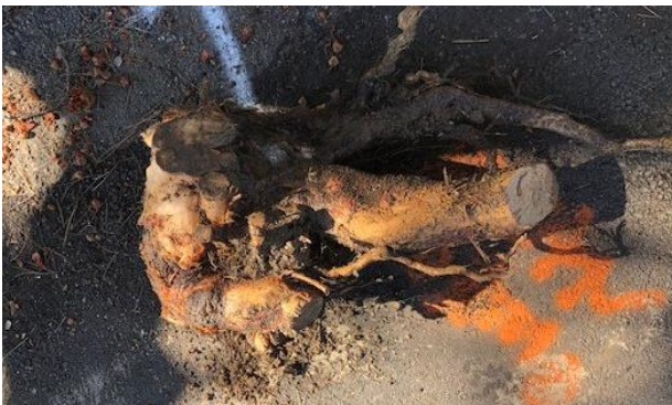
Figure 8 Root around supply line on Warwick
