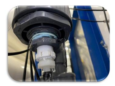
The pump and motor for MF train feed was sent in for repair. The pump had become very noisy; a bearing failure is suspected to be the cause of the noise and increased temperature while operating. Operators from Wastewater department assisted in moving the ¼ Ton pump and motor.
