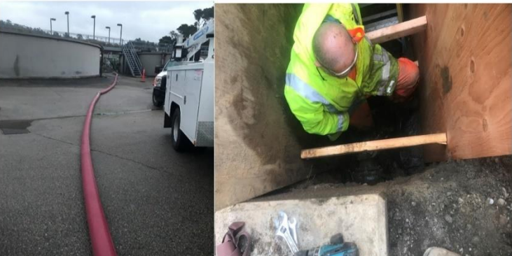
Figure 3 (Left) Lay flat hose crossing the plant (Right) Operator Artho repairing a broken influent valve at the grit chamber
