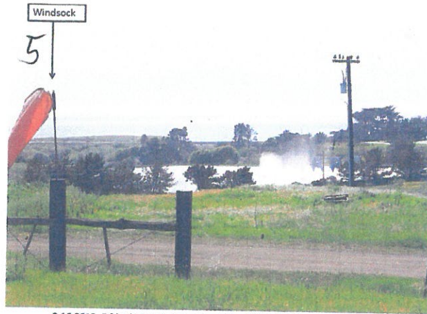
3-16-2015 Fifth photo taken in series of the CCSD EWS blower.
