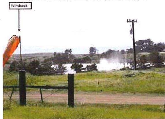
3-16-2015 Fifth photo taken in series of the CCSO EWS blower.
