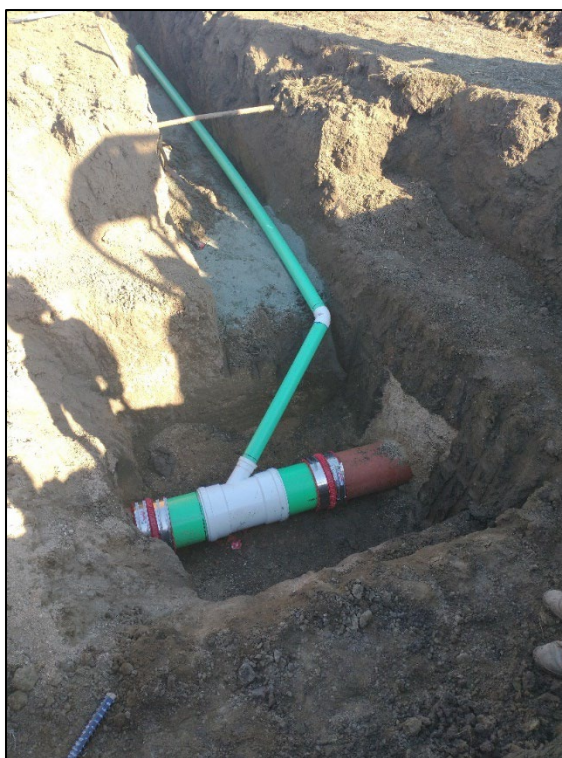
2. East Ranch Restroom sewer connection and lateral
