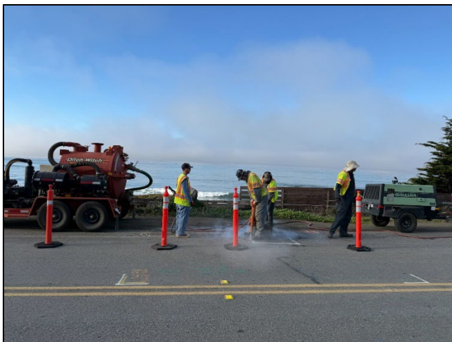
9. Moonstone Beach service line repair
