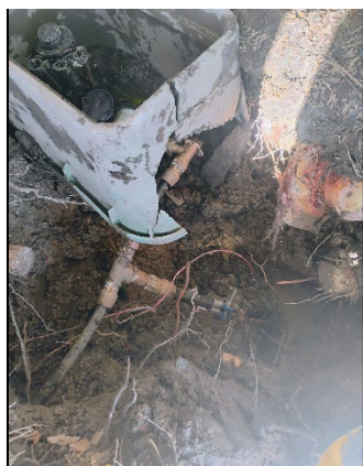
10. Service line repair
