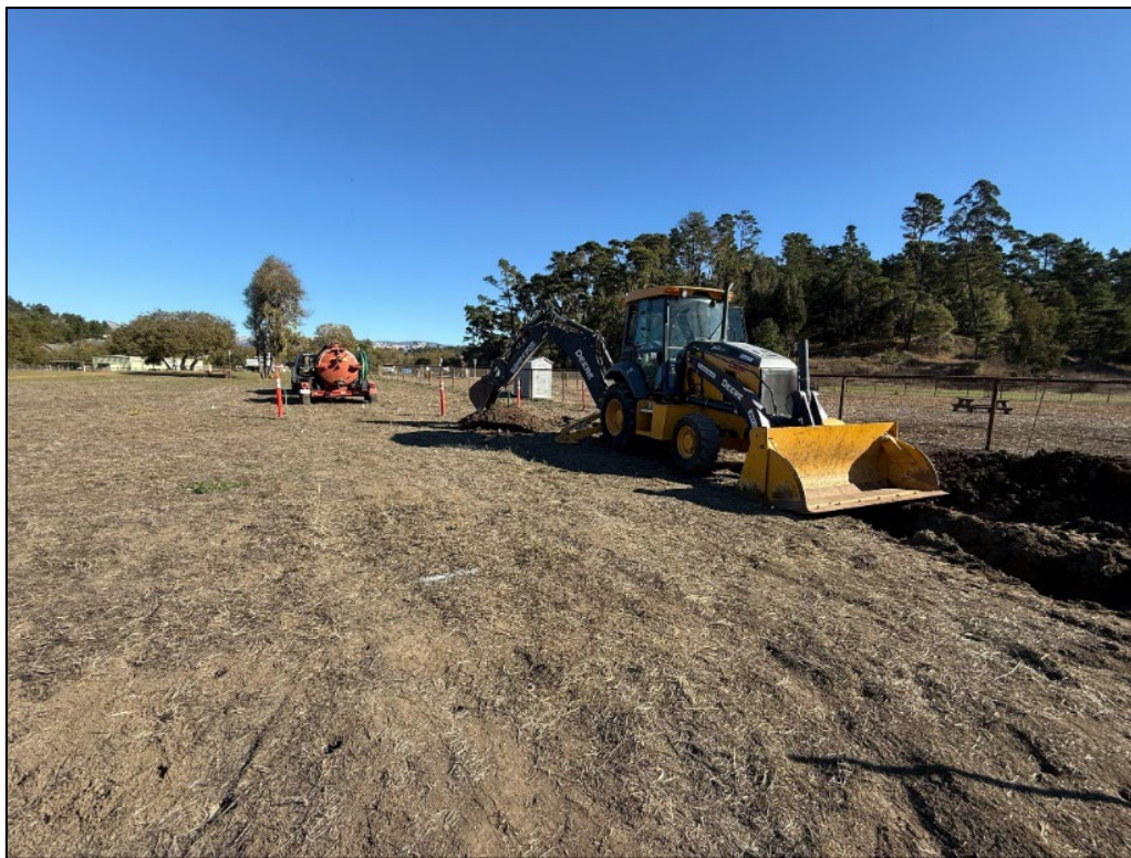
3. East Ranch Restroom water service installation
