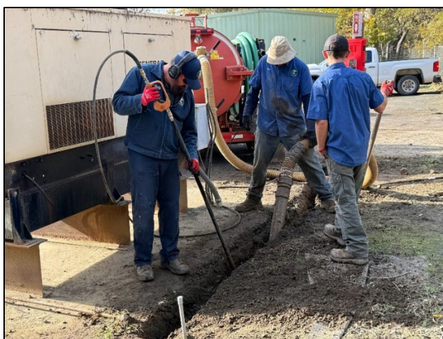
6. Soft excavation of the new electrical conduit trench
