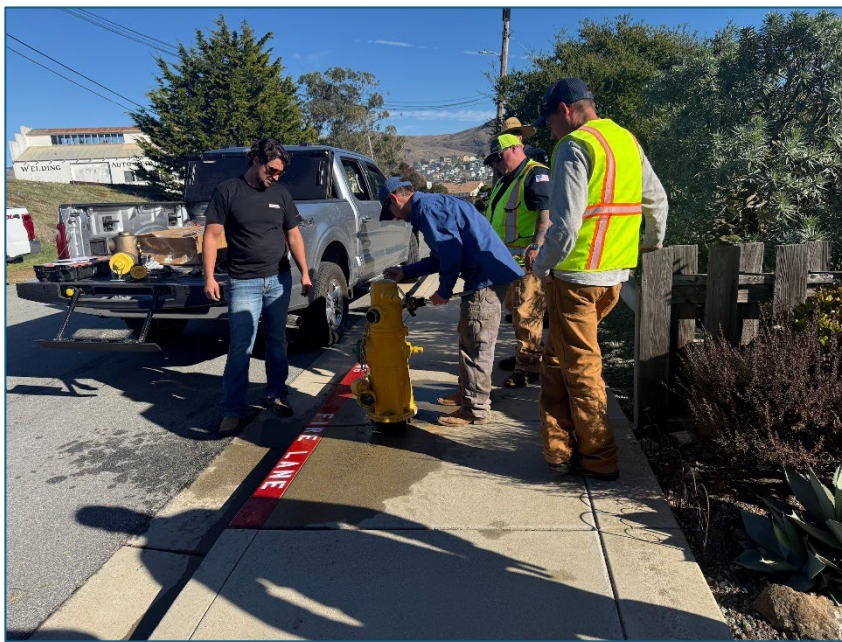
12. Hydrant gasket replacement training
