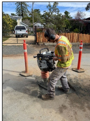
8. Recompacting post-repair
