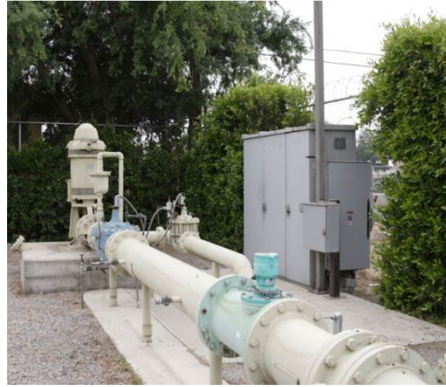
Figure 3.2.5-5 Wellhead of Typical Extraction Well
