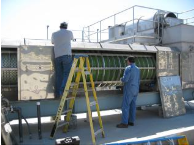
Press Screens being aligned with screw
