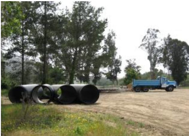
60-inch HDPE for Bridge & Center Street Property
