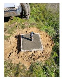
Also in January, the Air-Vacs on a reach of transmission main were replaced. The decades-old original parts were emitting high-pitched tones signaling end of life. An Air-Vac is used to release air from the pressurized distribution system upon system start-up and when pumps cycle on and off.
