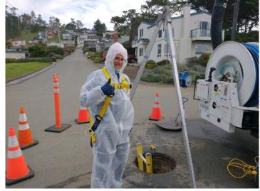
Figure B - Operator Toni Artho in full PPE for confined space entry
