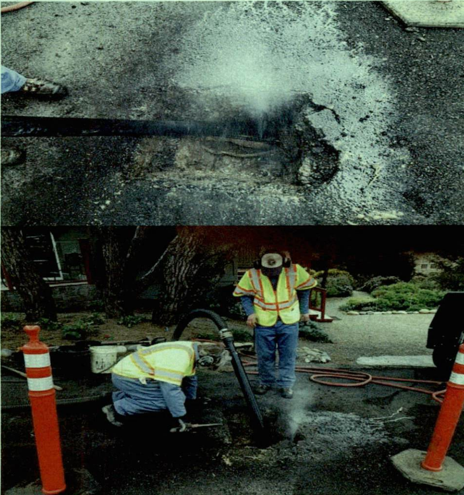
February 25 Service Line Repair at Ashby Ln/Warwick St.
