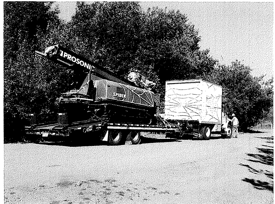
SIZE OF RIG WITH TRAILER AND TRUCK (168' SIZED RIG DESCRIBED IN GEOTECH#1 WAS DOWNSIZED)
