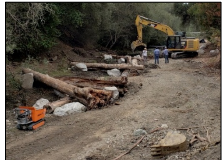
Construction of streambank restoration project in Santa Rosa Creek.
