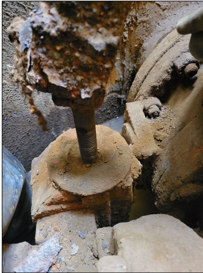
Figure 2: Operator Stem Assembly Close Up
