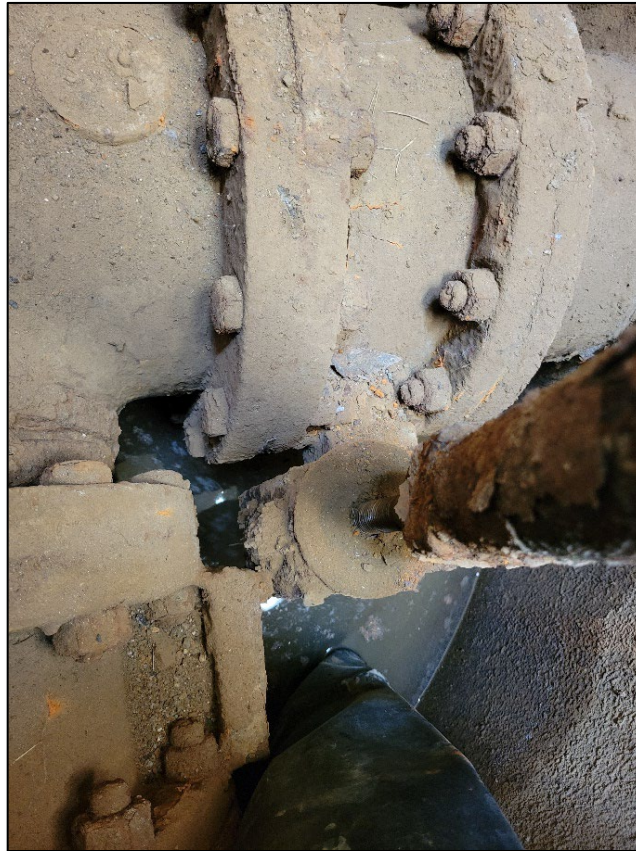
Figure 1: Operator Stem Assembly
