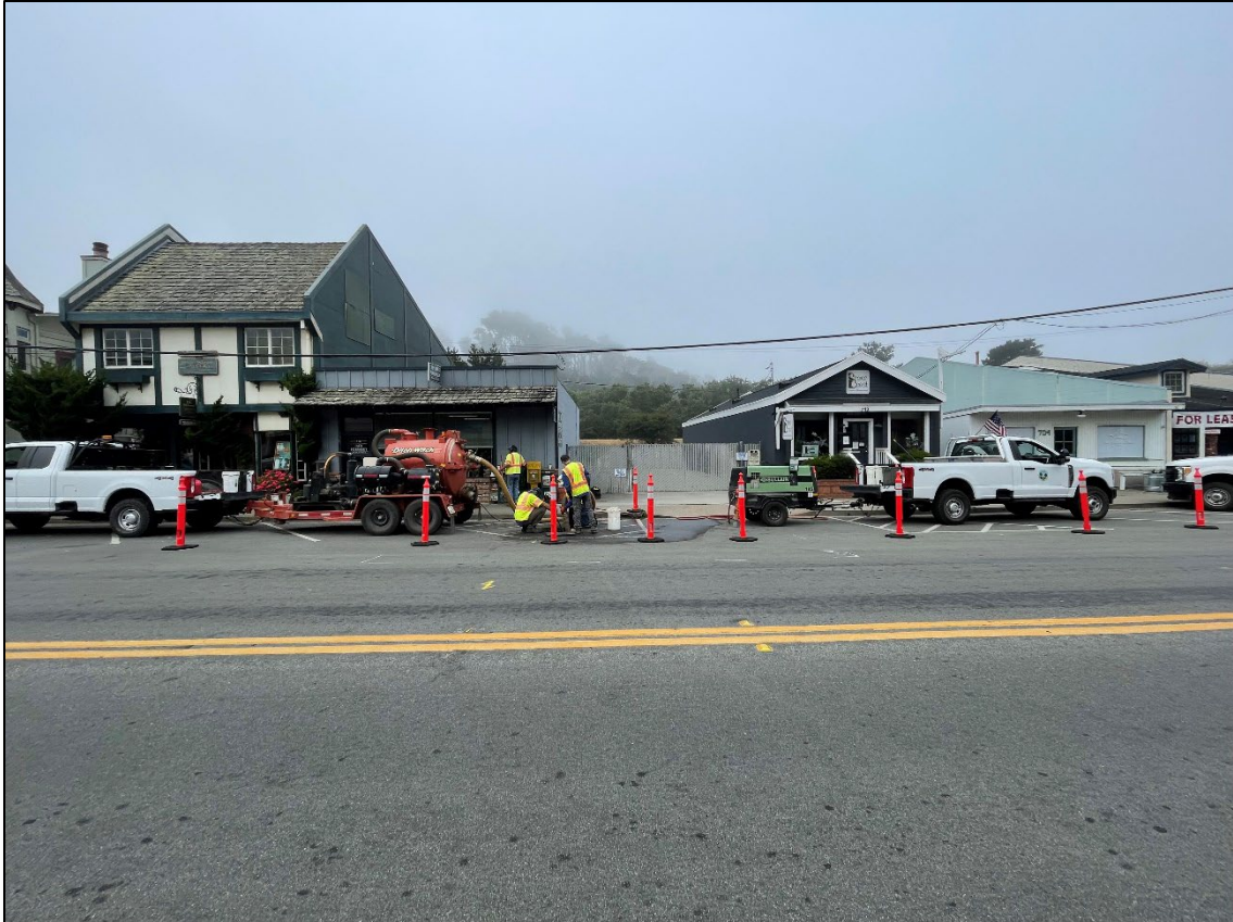
Figure 18: Area Along Main Street During Repair
