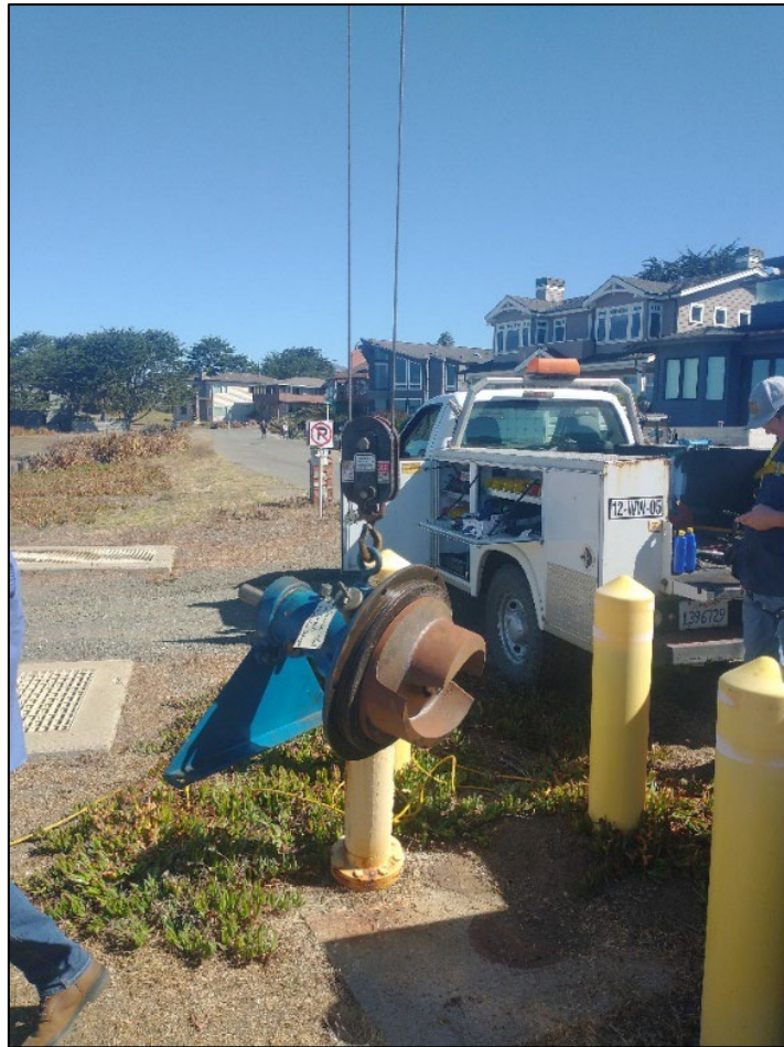
Figure 10: Maintenance at Lift Station A
