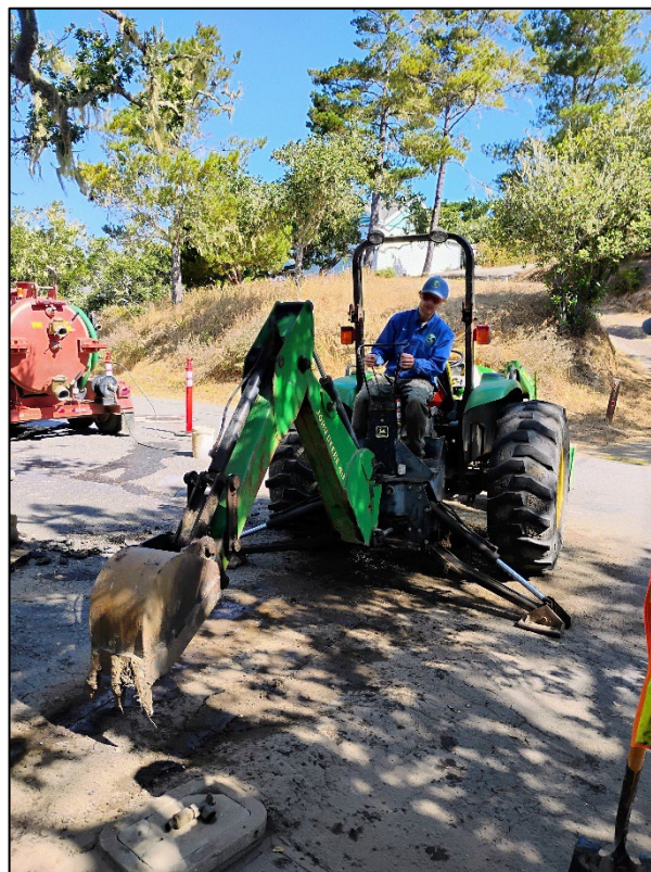
Figure 20: Main Street Repair and Replacement
